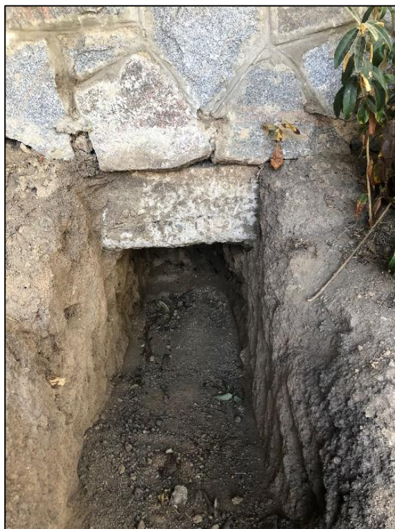
Plate 3: TP1 (Looking south).
