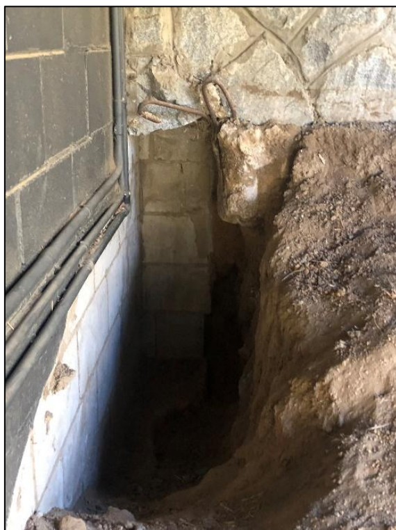
Plate 4: TP2 (Looking south).
