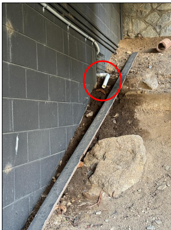
Plate 2: View looking south showing PVC pipe.
